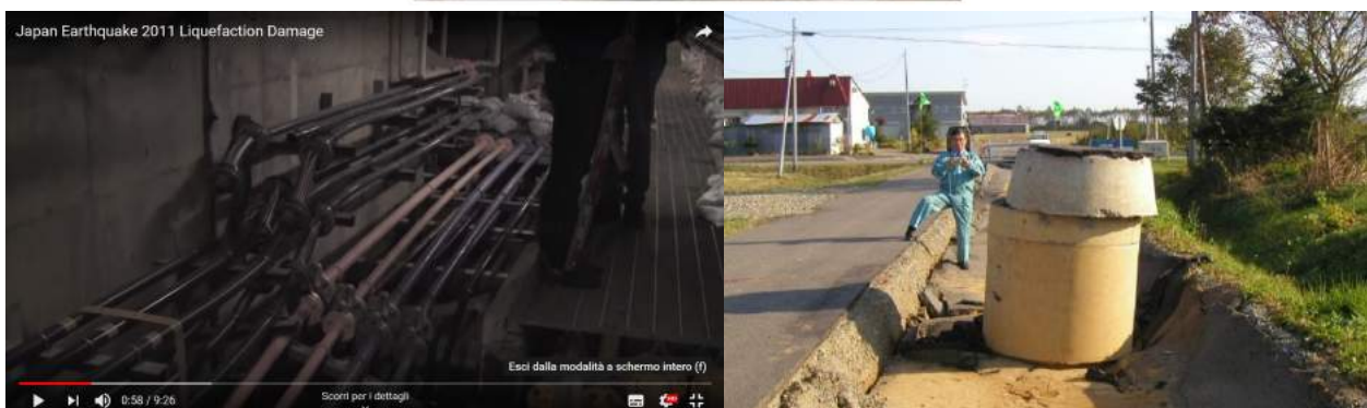
Figure 1-7: Liquefaction damage on water distribution and sewer system.
