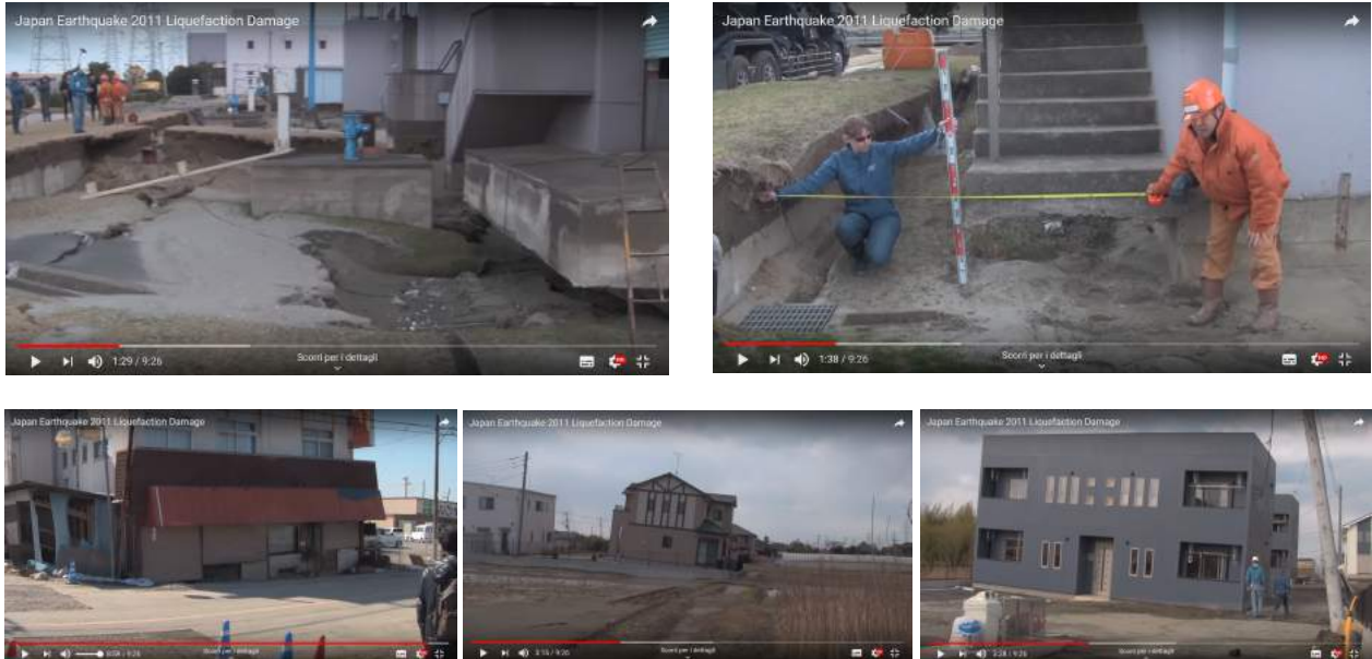
Figure 1-4: Uniform settlements, deflection and tilting of buildings caused by liquefaction (OSU, 2011).
