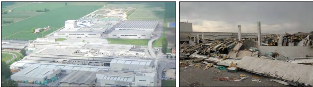
Figure 5-25 Example of industrial buildings in the district of S. Agostino and observed collapse.
