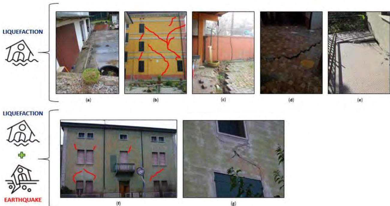
**Figure 4.3:** Damage induced by liquefaction
