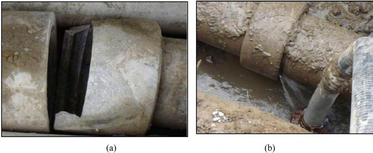
**Figure 5.47:** (a) Compression effects in AC pipe joint, Sewell Street Kaiapoi, (b) Tension effects in AC pipe joint, Sewell Street Kaiapoi (Reproduced from Toprak et., 2017)
