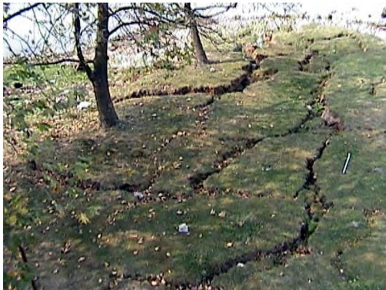
Figure 3.62: Ground displacements in the will (embankment) (Cetin et al. 2004).
