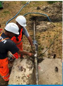
according to the "U" shaped path, then each hole was reamed withdrawing the drilling rods, and finally replaced in place by the final piping. The installation sequence was properly studied in order to maintain relatively "virgin" ground conditions on site.
