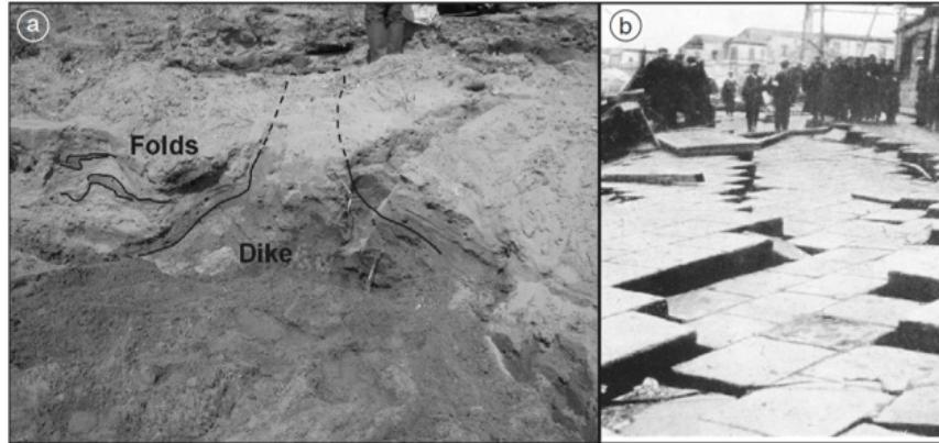
**Fig. 2a,b.** Examples of liquefaction features in Eastern Sicily: a) surveyed by means of paleo-seismological analysis in the Catania plain (after Guarnieri *et al.*, 2008); b) from historical reports, liquefaction in the Messina harbour after the 1908 earthquakes (after Baratta, 1910).
