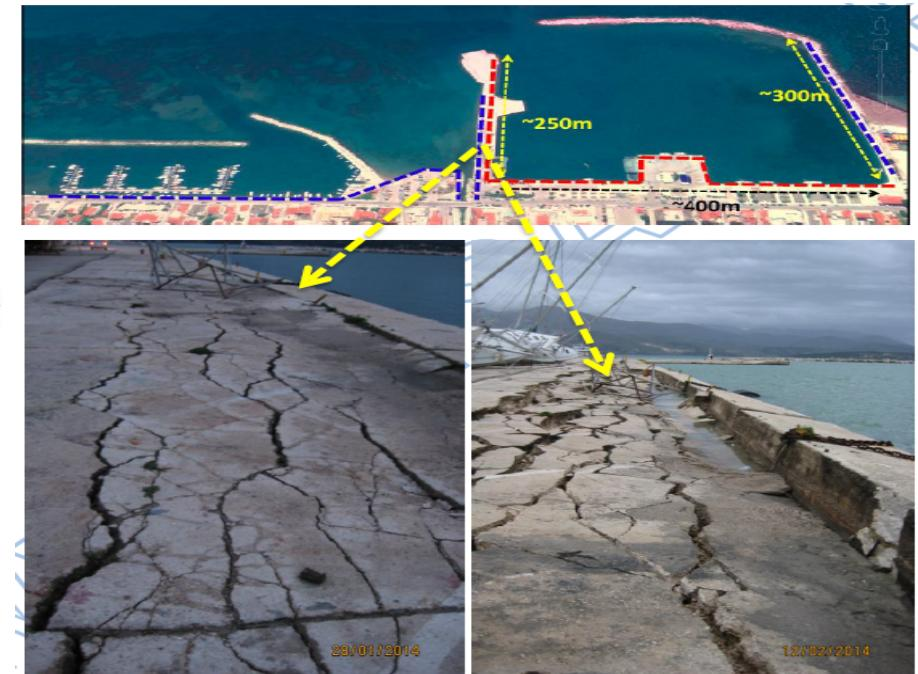
Liquefaction at Kefalonia port [Earthquakes report 2014]
